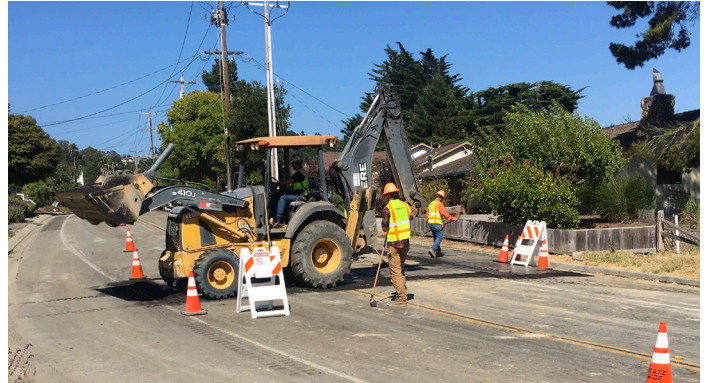
Water main replacement work on Clubhouse Dr.
