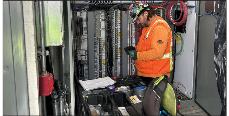
Electrical work at the Chanticleer Water Purification Center.
