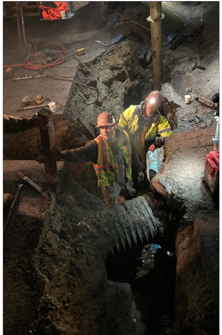
District Operations and Maintenance team making an emergency repair.
