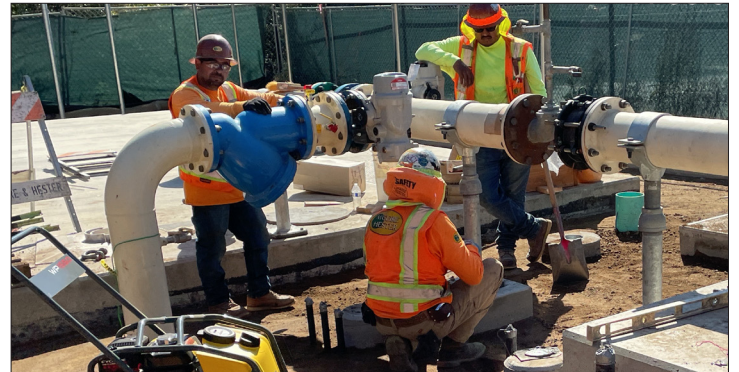
Willowbrook recharge well equipping.
