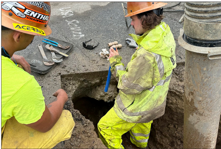
Our O&M team making repairs.
