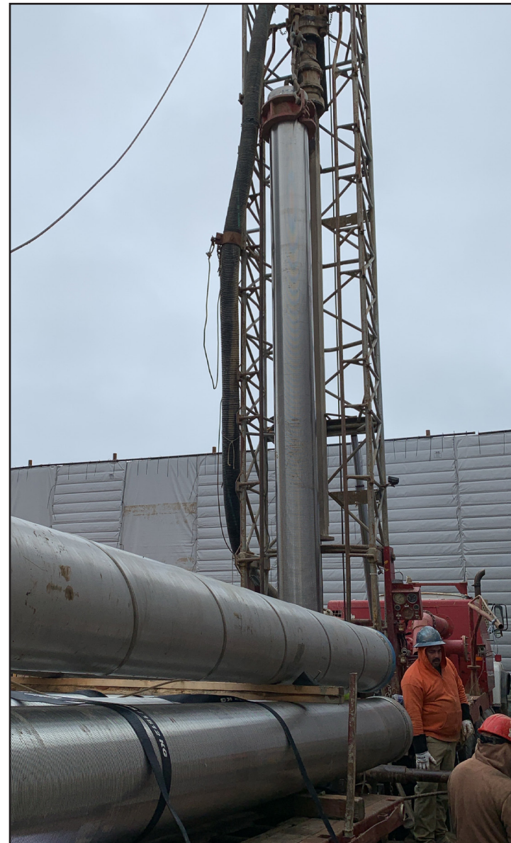
The new Country Club Well being drilled on Baltusrol Drive.
