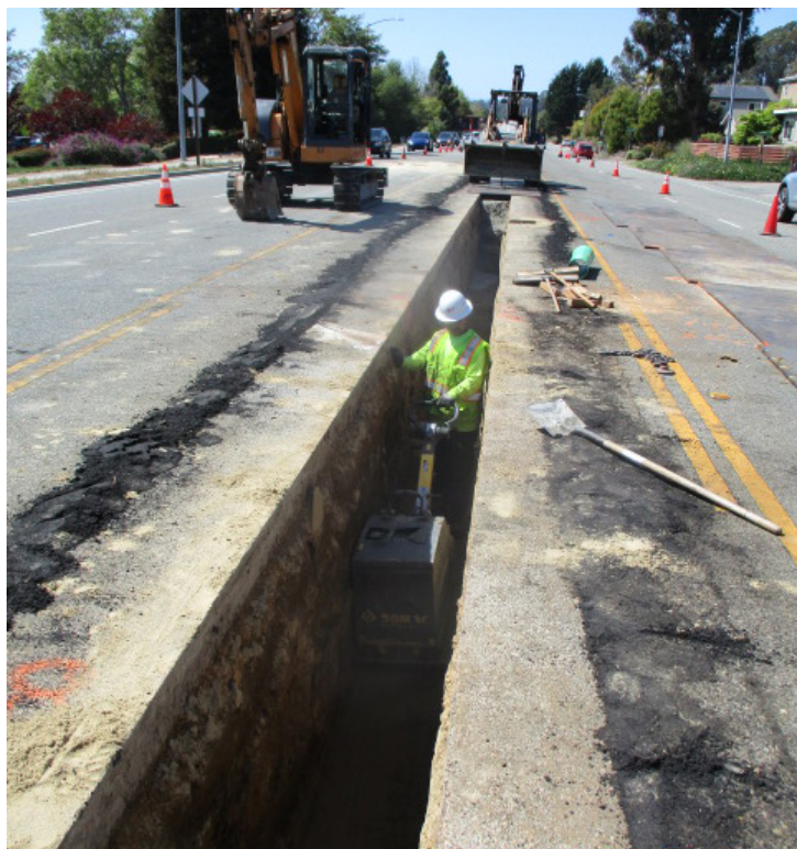
Soquel Drive main replacement.
