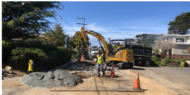
Bayview Drive main replacement.
