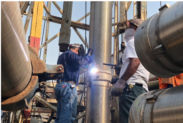
Welding of the well casing pipes.
