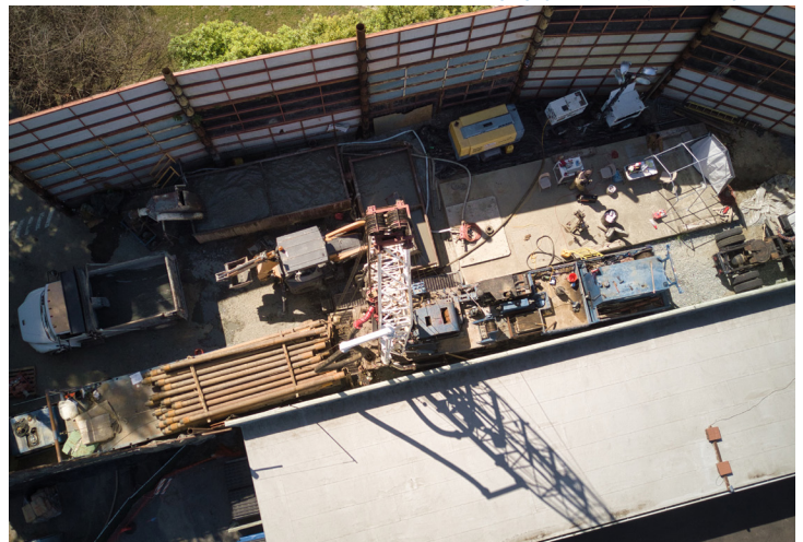
Aerial view of the Monterey SWIP Well site
