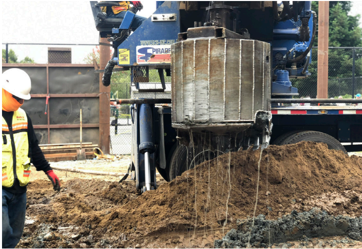
Drilling the initial bore hole.
