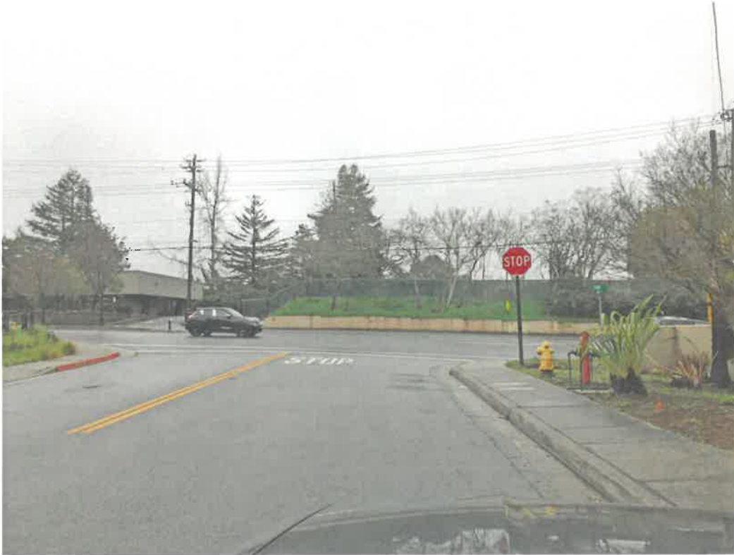
Existing view of Project Site
