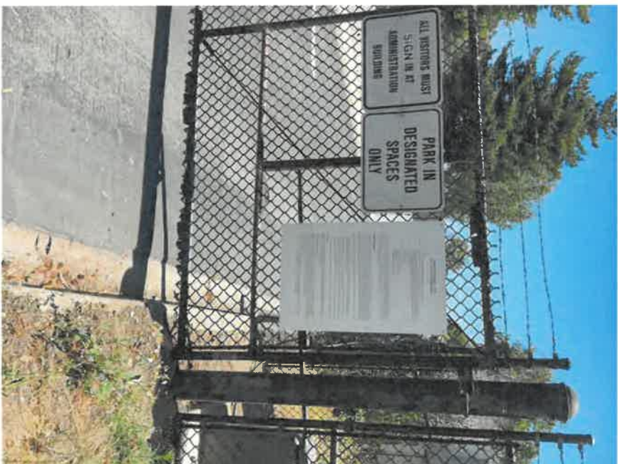
Photo 3 - View of SC WWTF Entrance Gate
