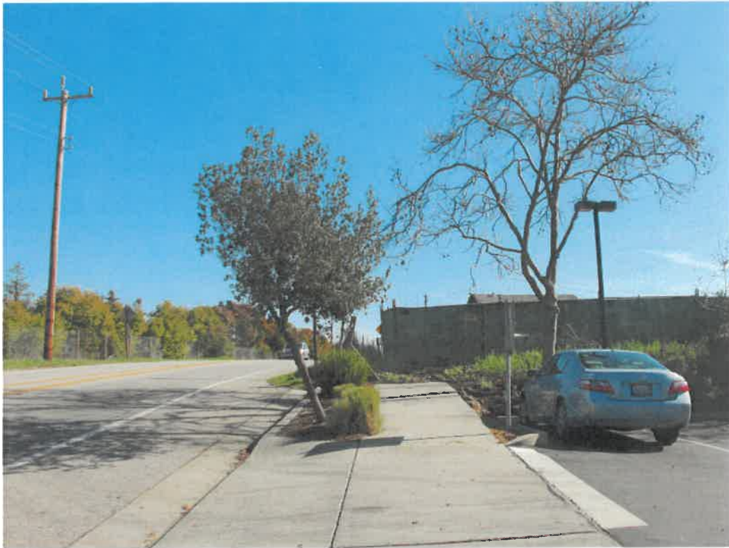
Existing view of Project Site
