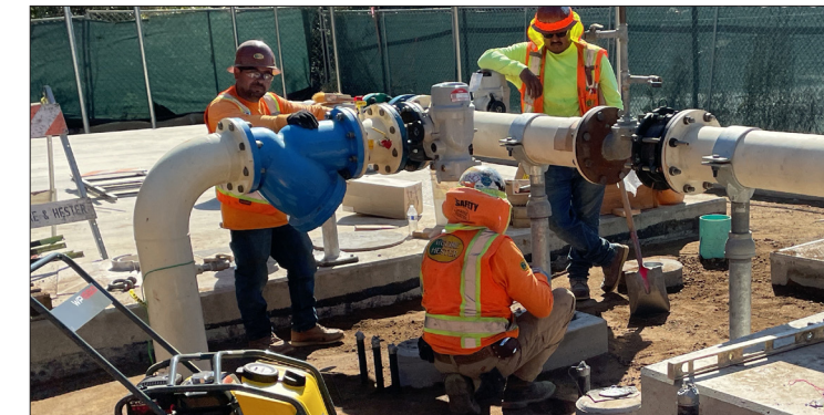
Willowbrook recharge well equipping.
