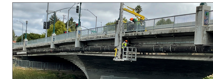
Conveyance pipeline being hung on the Laurel Street bridge.
