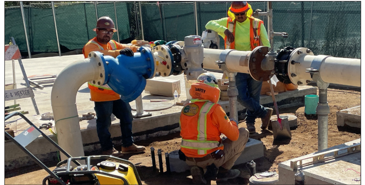
Willowbrook recharge well equipping.
