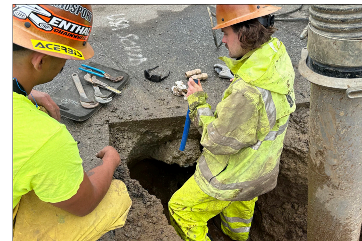
Our O&M team making repairs.
