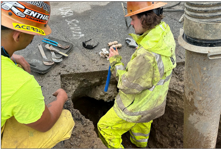
Our O&M team making repairs.
