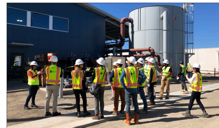
Community members on a construction tour of the Pure Water Soquel Purification Center.
