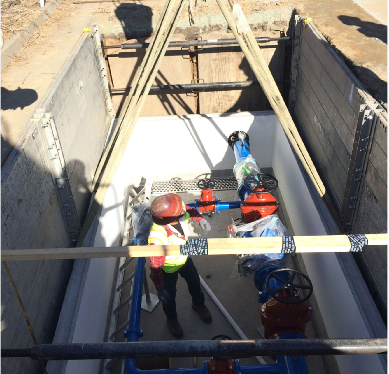
Photo of Underground Vault Installation on Sumner Ave. in Aptos
