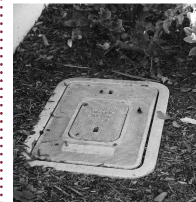
Maintaining appropriate clearance around the meter box allows District staff to read, service, and repair the meter.
