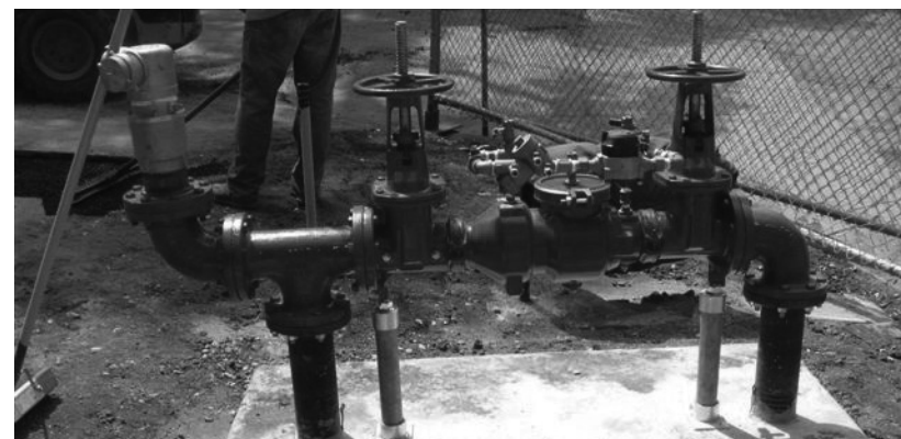
State law requires water suppliers to protect their water systems from contamination or pollution through the use of backflow prevention devices.
